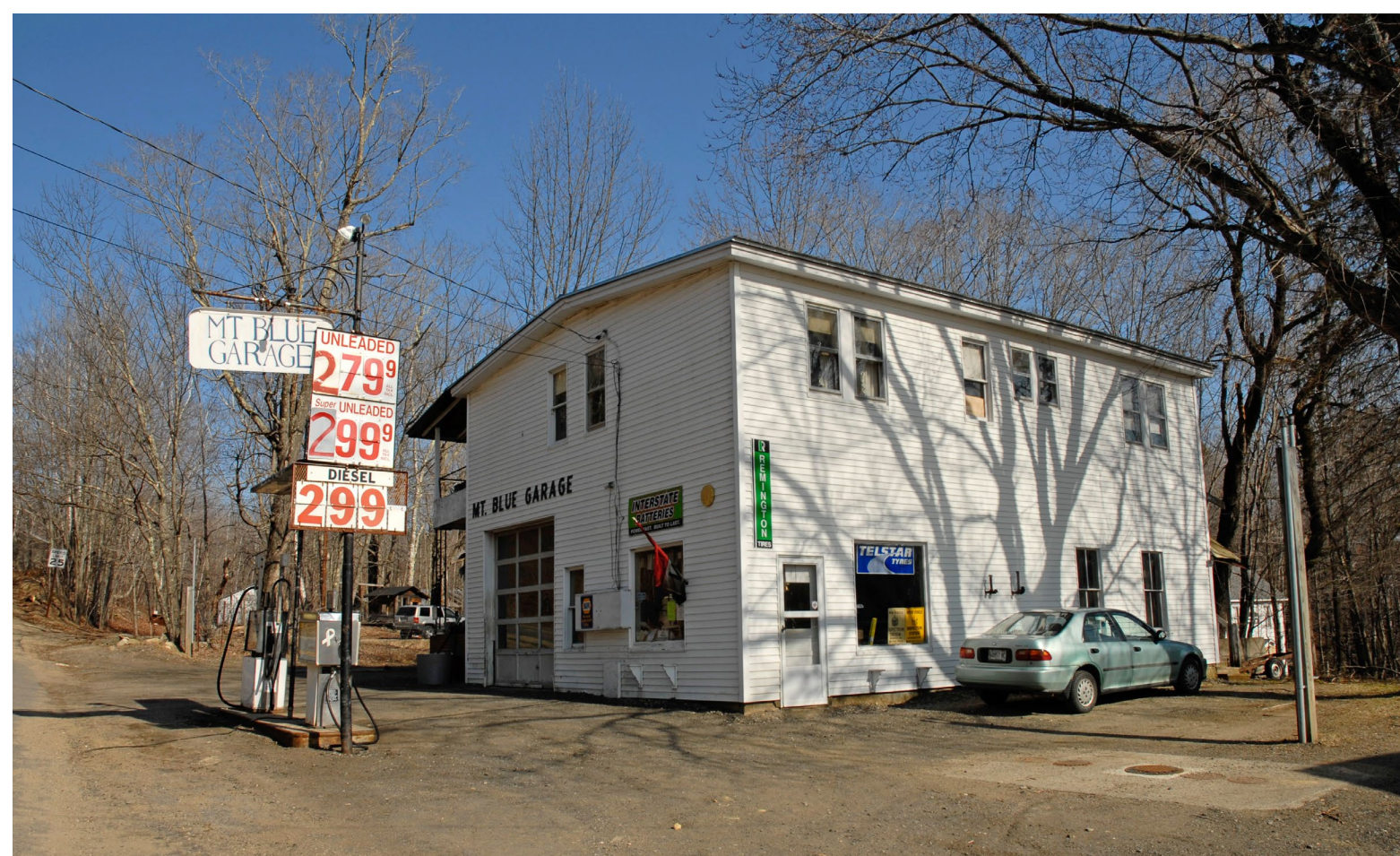
5: Mt. Blue Garage, Weld, ME.
