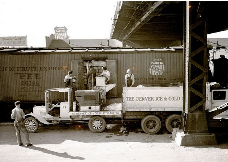
21957 -- Link-Belt Ice Slinger re-icing hampers of peas at the Denver Ice and Cold Storage Co., Denver, Colorado. October, 1936.
