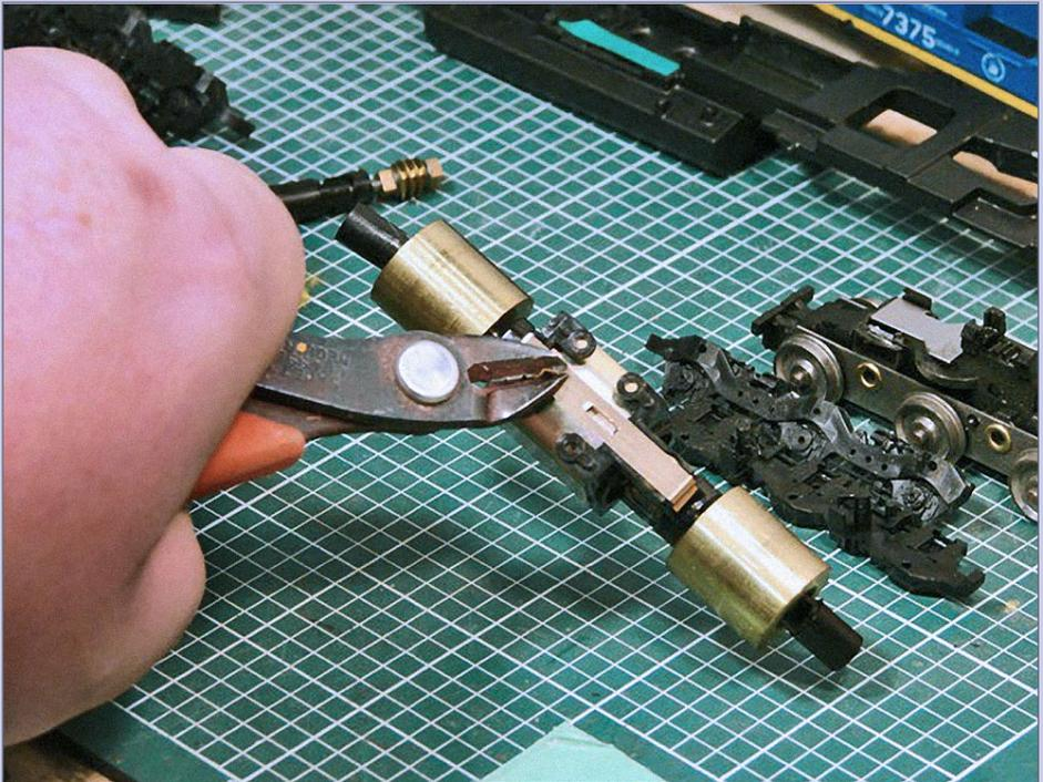
**34. Remove prongs:** Cut off the prongs on the bottom motor clip.
