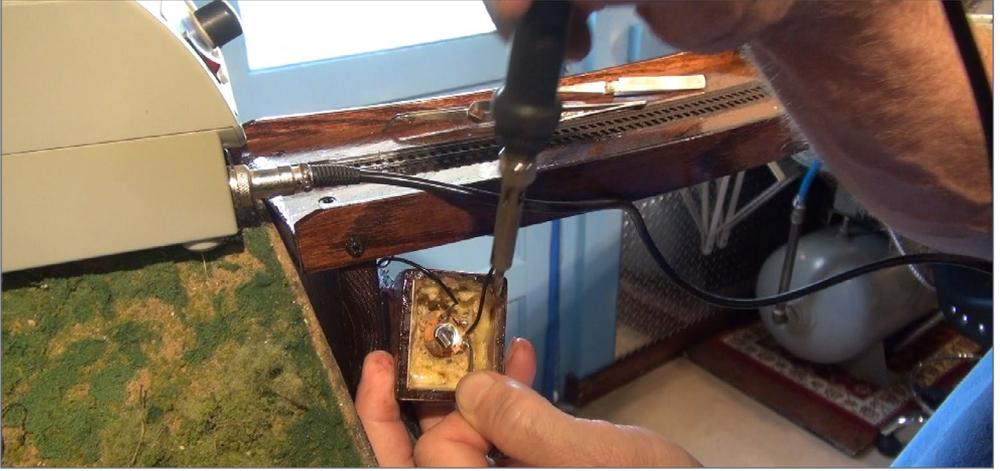
12. I drilled two holes in the lift-out section to run power wires from the rails through the  $\frac{3}{4}$ -inch plywood, feeding the wires into the small wood box and soldering the leads to the microphone jack solder tabs.
