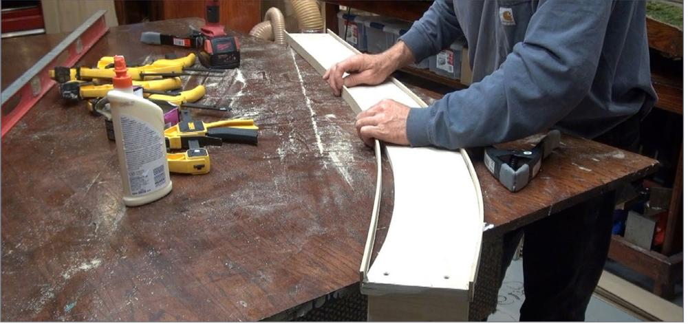
8. Moving back to the workbench, I cut two strips of  $\frac{1}{4}$ -inch plywood to form protective walls  $\frac{3}{8}$ -inch-high along both sides of the main. This was glued with wood glue and screwed in place with  $\frac{3}{8}$ -inch metal screws.
