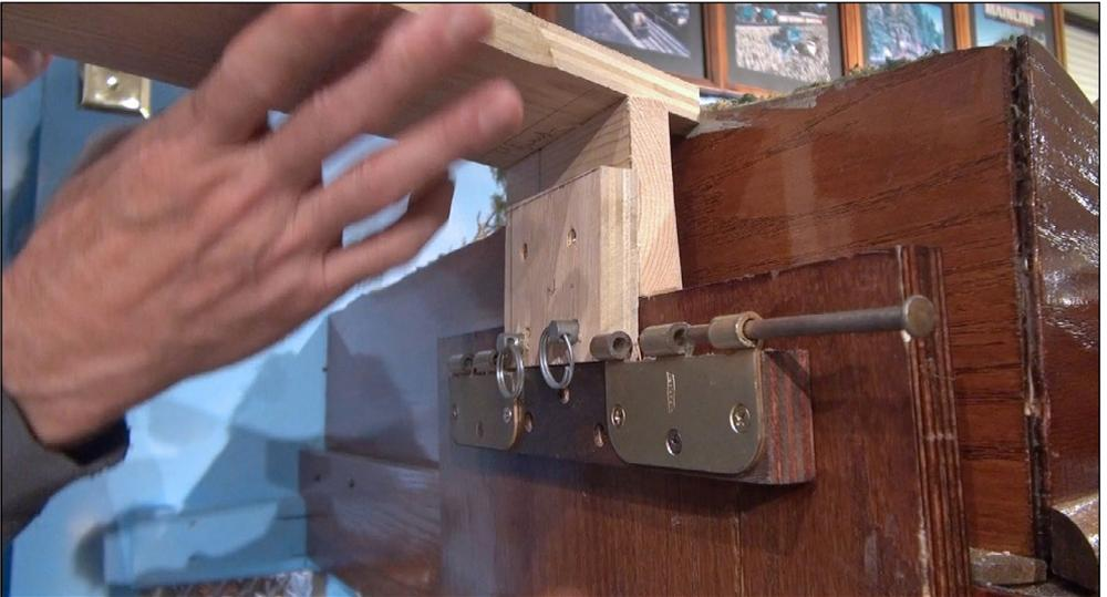
7. These pins fit through the holes, making for a very solid attachment point to the existing stained 3/4-inch plywood fitting between the old door hinges. The pins easily pull out with the help of a metal ring pull that your finger fits into.
