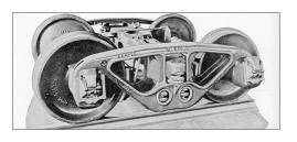
A unique trunnion design kept the bolster and side frame in alignment, and eliminated the need for a heavy transverse spring plank that could weigh up to 300 pounds. Spotting features of National B trucks are the end pocket in the bolster that keeps the spring group in position, and the pair of round holes in the side frame. Some National B trucks were later fitted with roller bearings.
