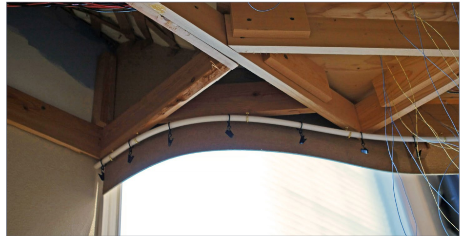
15. When MRH/TMTV visited Jeff Sargent’s layout in 2015 to shoot a layout story, Jeff showed us his clever system for attaching layout skirting. Notice the cup hooks, the ½” white flexible water hose, and the sliding 1” shower curtain-style clip rings. The SL2 module section design accommodates this system to attach skirting.
