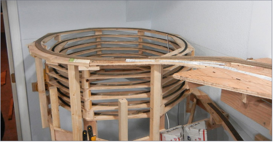
12. The helix in the alcove entering Parker Yard, to the right. Radius is 18" with a climb of 2-3/8" per loop.
