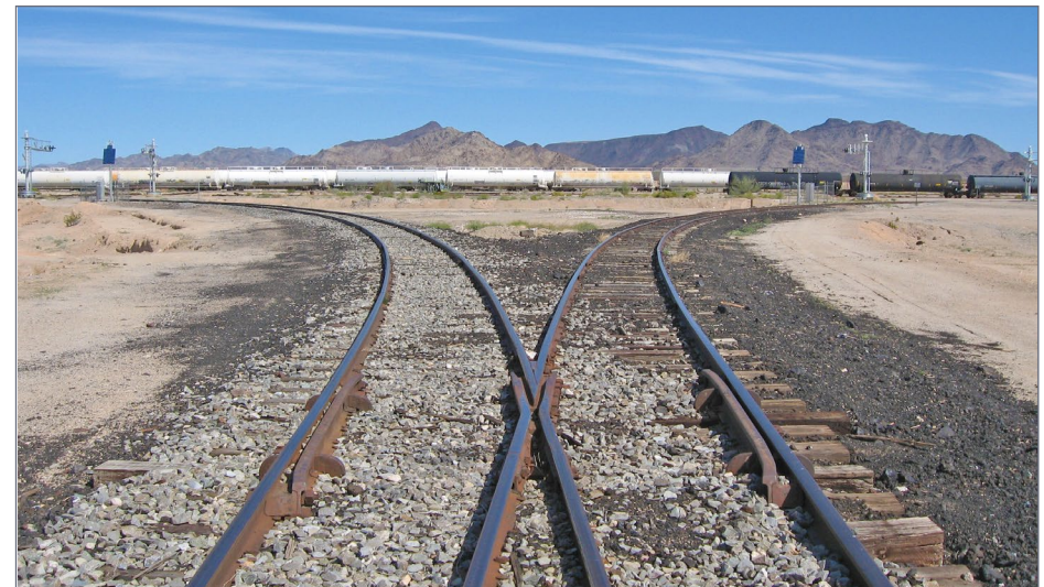
7. Tank cars of anhydrous ammonia sit in Rice at the wye switch leading to the Blythe Branch. KL Smith
