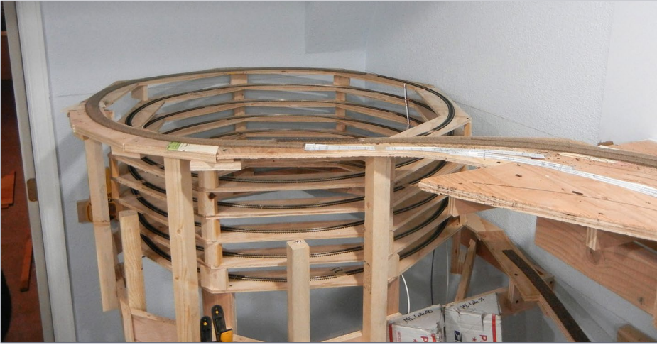
12. The helix in the alcove entering Parker Yard, to the right. Radius is 18" with a climb of 2-3/8" per loop.
