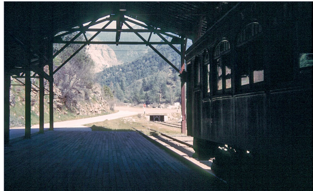
26. This was the view from the passenger loading platform under the train shed looking toward Yosemite Valley which was nine miles further east. De-training passengers enjoyed this view for 38 years. The equipment loading ramp is visible near the highway. Al Rose photo
