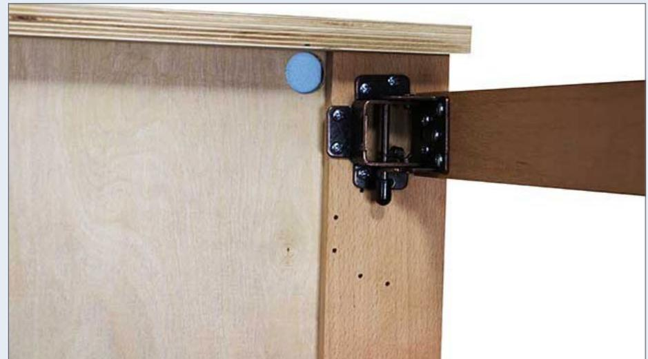
16. (Left bottom) This photograph from Kam Konnect shows how a dropdown module is built with 18mm Baltic Birch (13 plies thick, total 3/4") plywood sides and ends. The base is 1/4" hardboard with 1/2" foam board for scenery. I will add 12mm (1/2") cabinet-grade plywood for the track roadbed.
