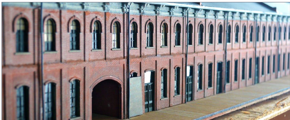
18. The back side of the station shows the improved drain pipes and some blanked-out window and door openings. Photos made at this stage are a good way to spot flaws to correct before final assembly. I really like the look of the station all boarded up.
