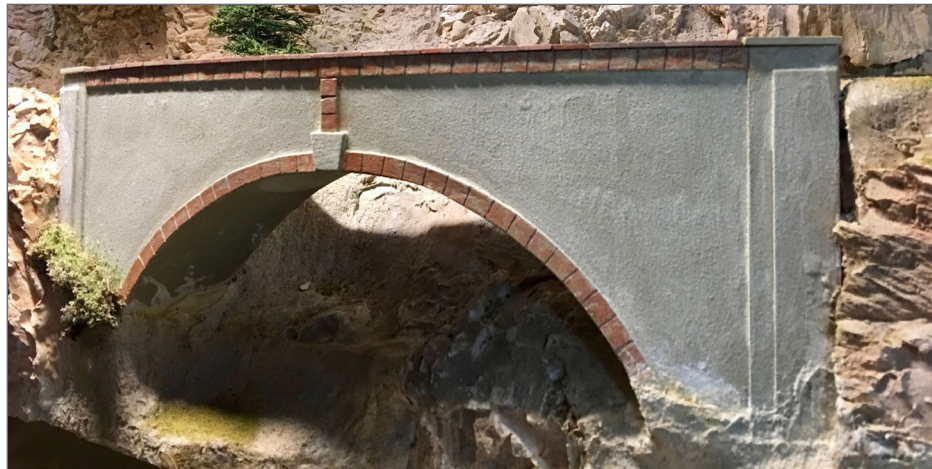
8. Ken Schei's Calumet and Hecla RR On3 layout has an amazing collection of bridges and rock work. Bruce Petrarca photo
