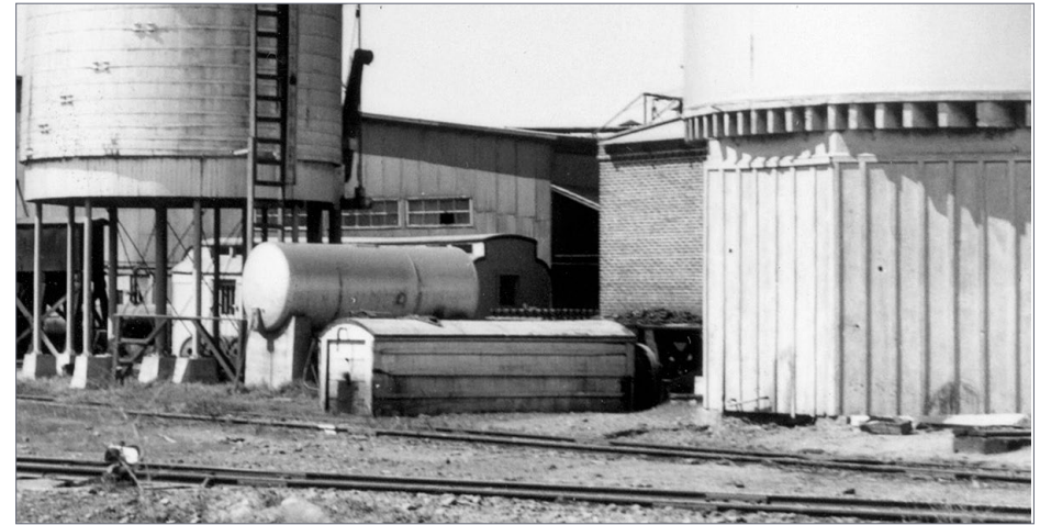
19. The long item on the right next to the oil tank was the electric pump that pumped Bunker C from the settling tank into the oil tank. I believe the round tank left of the pump used to store gasoline for the speeders. Jim Boynton photo
