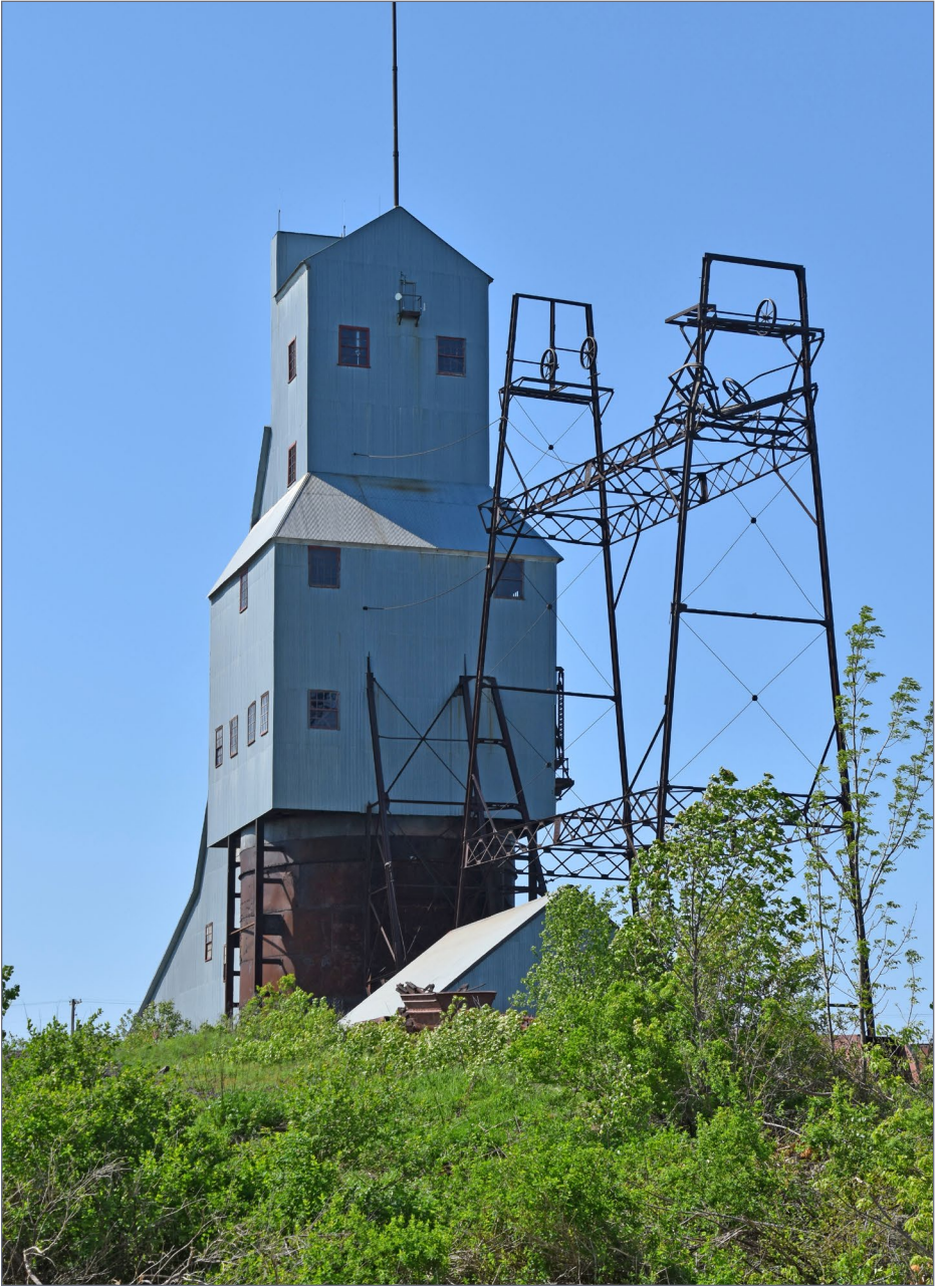
21. Quincy mine No. 2 shaft head house.
