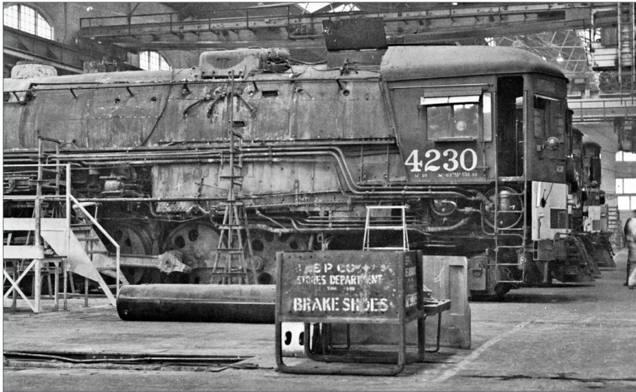
16. This 1955 view inside the Erecting Hall at Sacramento General Shops shows cab-forwards undergoing class repairs. In the foreground is a skid for brake shoes, labeled "SP CO STORES DEPARTMENT," as well as indicating the desired contents. Ken Yeo photo, Bob Church collection
