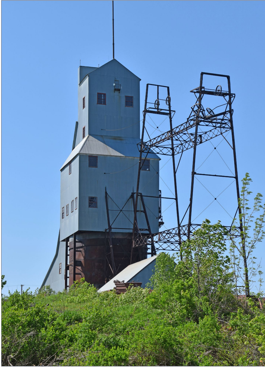
21. Quincy mine No. 2 shaft head house.
