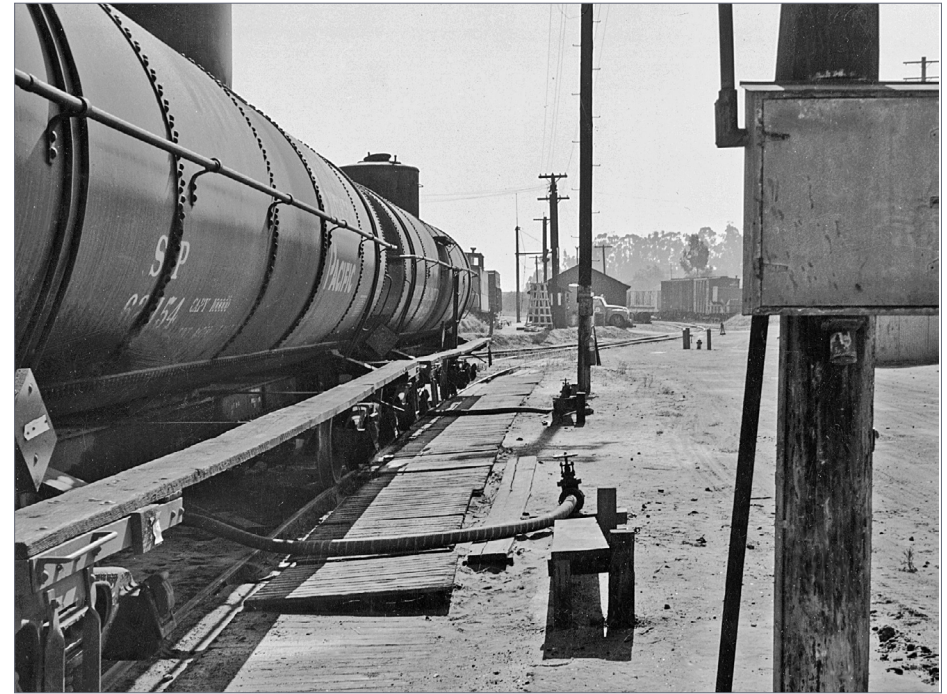
6. This is the SP fuel track at San Luis Obispo, CA in the late 1950s. Hoses are connected to the tank cars for gravity unloading. The duckboards for workmen alongside the track are evident. Southern Pacific photo
