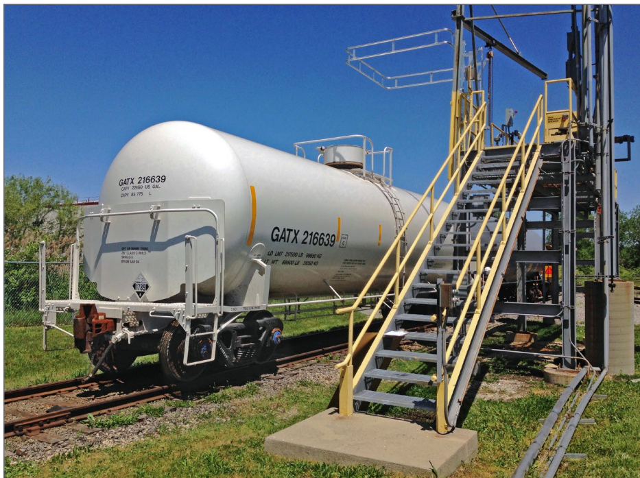
2. An excellent example of simple unloading rack in a small transloading facility. Chlorine Institute photo
