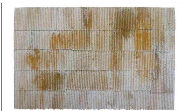
49. Completed corrugated siding.
