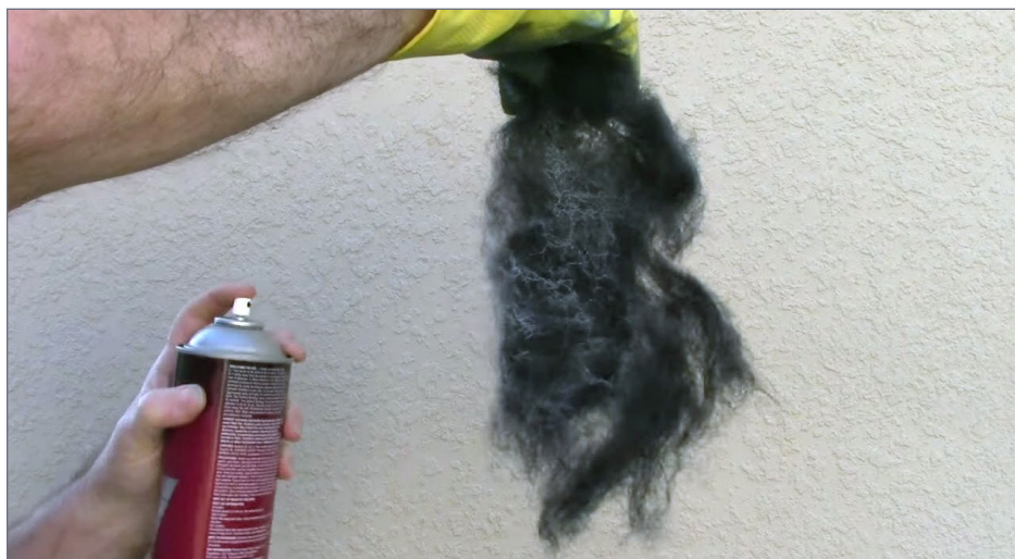
4. Applying adhesive to the poly fiber.
