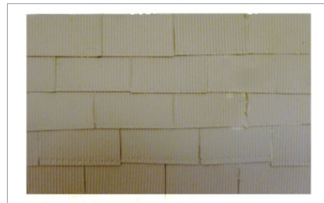
47. Spray paint the metal siding light primer gray to provide a consistent base for weathering.
