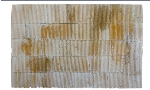
49. Completed corrugated siding.
