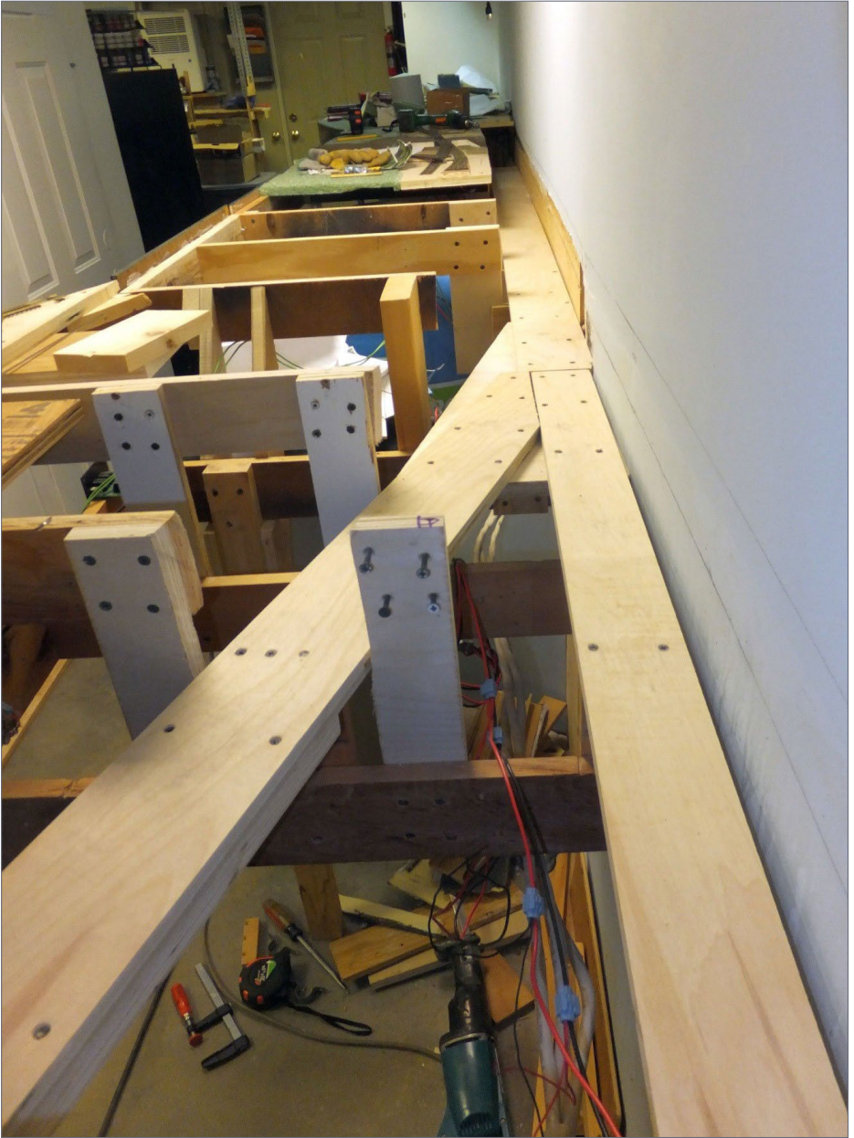
12. Ready for track! The new pathway to the lowered staging yard is in place below Ransom and Tunkhannock.
