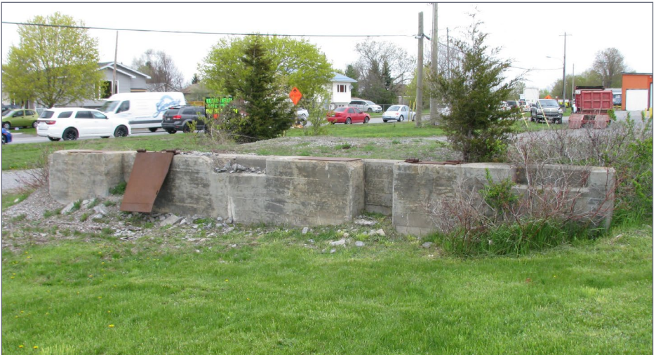
18. The concrete TOFC ramp at Belleville, Ontario will probably stand long after the trucks that it served have rusted away.
