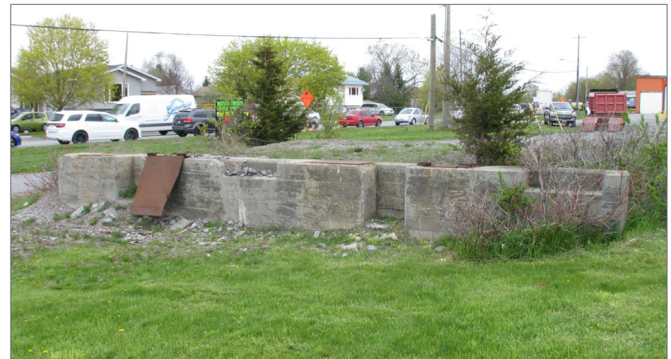
18. The concrete TOFC ramp at Belleville, Ontario will probably stand long after the trucks that it served have rusted away.
