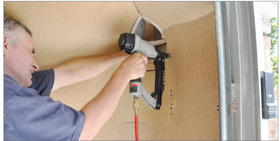
12. My air nailer is a handy tool for doing small pieces like this. If you don't have a nailer, screws will work also.
