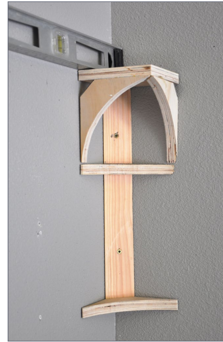
7. The corners were installed first, then I leveled the top of the backdrop using them as my height guide. The spine of the corner pieces are sections of 2x4 that I ripped at a 45° angle and attached to two of the curved pieces for the cove.
