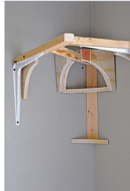
8. I added the brackets and extensions adjacent to the corner pieces, plus some additional cove pieces so there is plenty of material to screw the Masonite into.
