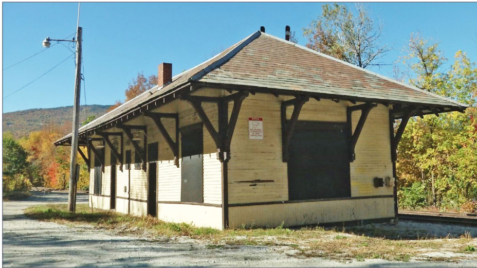
2. The depot at Ludlow has avoided the wrecking ball.
