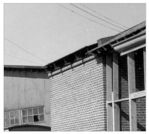
12. A close-up of the previous photo clearly shows the 8"-tall I-beams mentioned in the 1917 Inventory as well as the brick relief on this side of the building. The 2x4 wall construction of the adjacent breezeway is also visible. *Al Rose photo*
