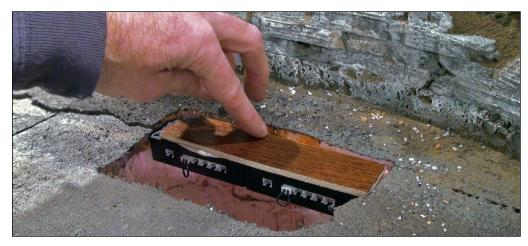
15. The two light hubs will be glued flush in the foam facing down so I will have access to the potentiometers with a long screwdriver when it comes time to adjust the lights' brightness.
