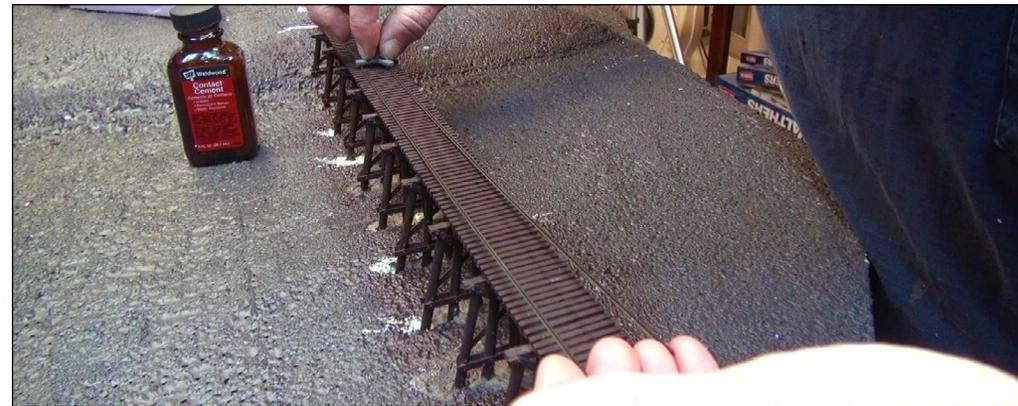
44. I glued the track to the roadbed with Liquid Nails. I glued the rail to the bridge deck with contact cement keeping everything in gauge with Micro Engineering HO scale three-point track gauges. I further attached the rail to the bridge with scale track spikes pushed through the bridge ties with a pair of pliers. I attached 4x8 guard timbers to the outside of the rail, gluing these to the bridge deck.
