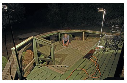
7. I sanded the train deck where the dogbone layout loops back – sanded it down to the bare wood with a six-inch orbital sander and 60 grit paper.
