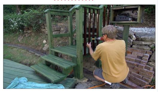
8. I applied a fresh coat of semi-transparent green stain to the deck. I stained the stair trim pieces with brown stain, and reattached accent wood to the deck.
