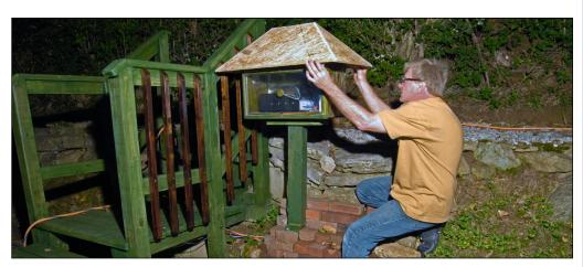
9. I built a waterproof box of wood on a pole, with a hip roof, to house the electronics and power supply. This was hidden under the deck before but I erected it on a pole for better radio reception with the hand-held radio controller.
