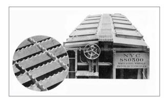
32. Apex Tri-Lok metal running board.
