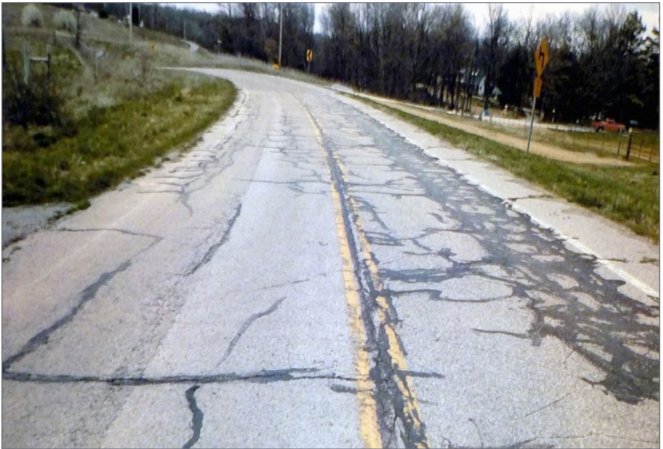
20. A section of the Old Hwy. 59, Siloam Springs, AR.
