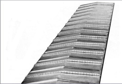
28. Modern Pullman-Standard roof from the 1970s.
