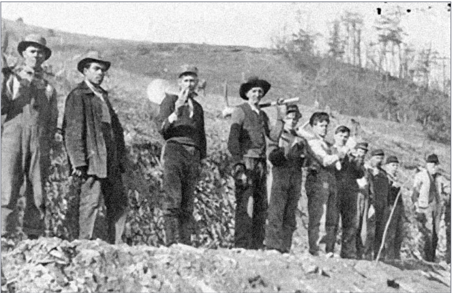
2. Construction of trestles on the TM&P and workers. From the internet, source unknown.
