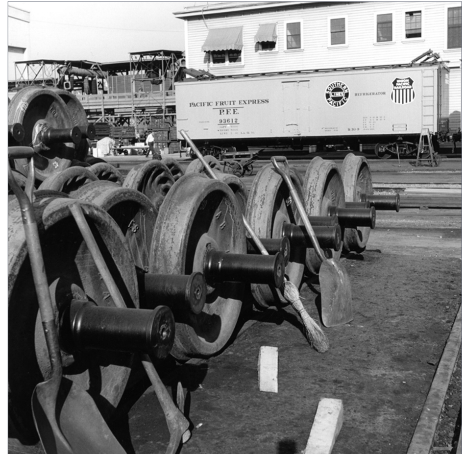
35. Many prototype photos show axle journals prominently, such as the photo, taken at PFE’s Los Angeles Shop in December 1950, showing two rows of wheelsets with the axle journals quite visible. These have been machined and coated to protect them. Note also that the wheelsets are on paired rails (see another pair at right), so that all will roll even in this double-stacked arrangement. The wooden wedges would be useful to restrain rolling. In the background, posed in front of the Shop office, is PFE 93612, a member of PFE’s largest car class, R-30-9. Richard Steinheimer
