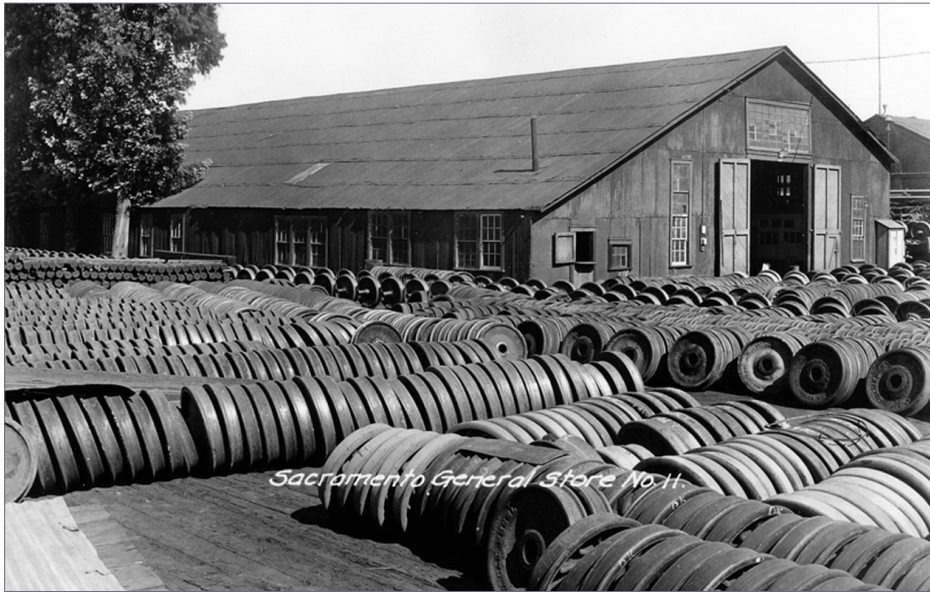
13. The wheel storage area outside Building 11 of the General Stores at Sacramento General Shops of the Southern Pacific. Wheels here are mostly new, but some rows of worn-out wheels can also be seen. A line of wheelsets is near the building. Southern Pacific photo X8351-04, John R. Signor collection
