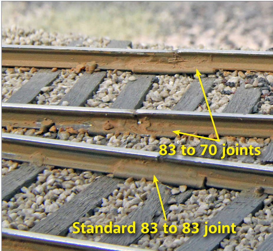
8. ME code 83 rail to code 70 rail joints using squished ME code 83 rail joiners, compared to a standard code 83 to code 83 joint.
