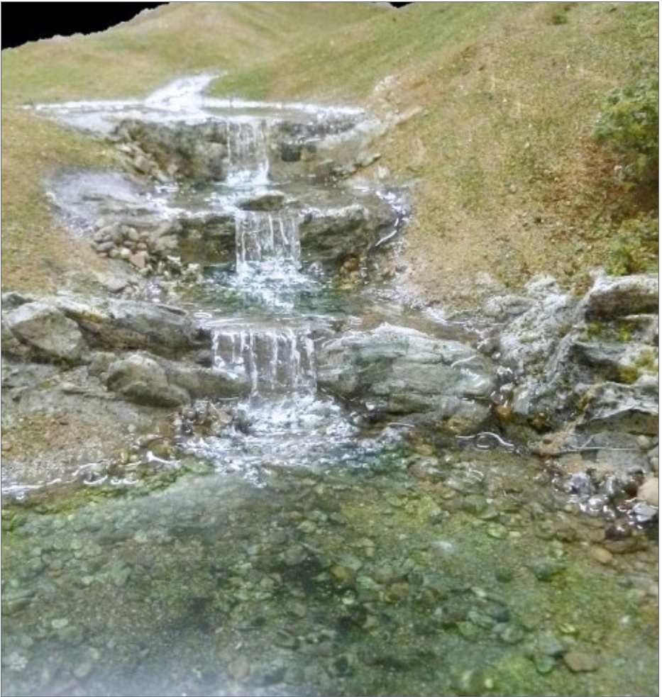
54. The completed Noel Branch water features.
