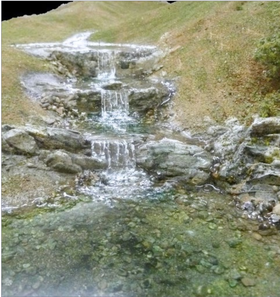
54. The completed Noel Branch water features.
