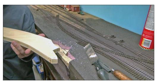
20. Gorilla Glue holds the plywood base into the foam on both ends of the lift-out section. After a test fitting came the final carving of the form for a perfect fit.
