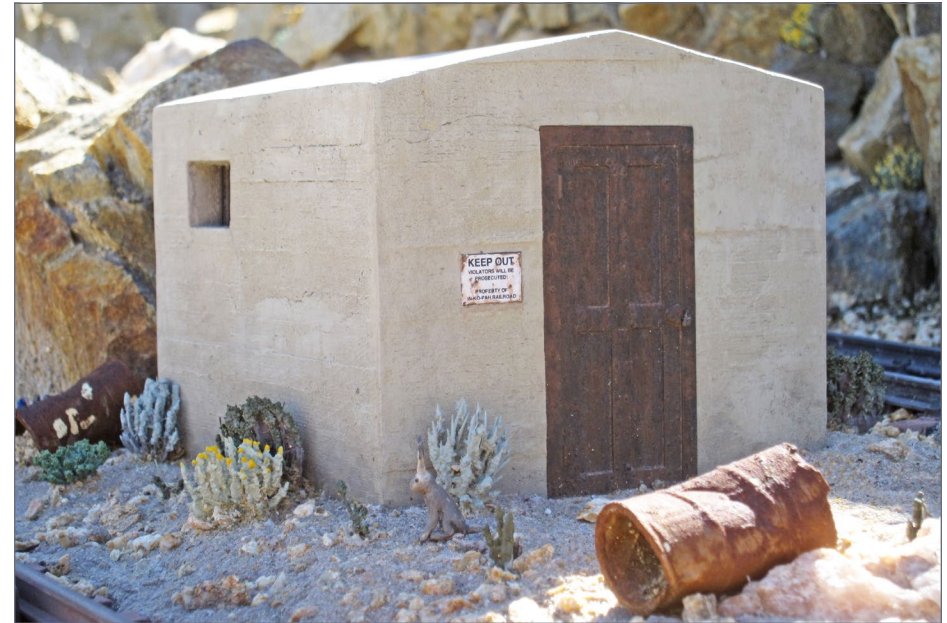
6. A former jail, this cast concrete building now provides storage for the railroad.
