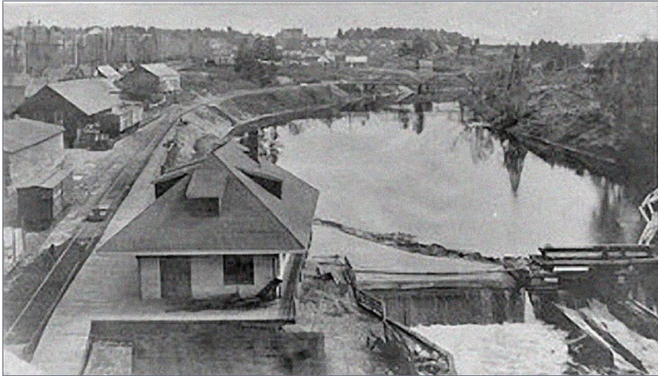
1. The station area of Pembroke, along the bank of the Muskrat River. The roundhouse is about ¼ mile down the track around the bend in the river. Author's collection
