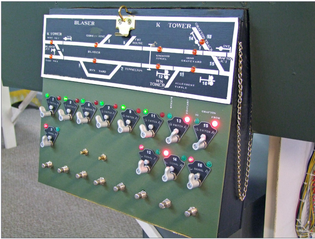
7. Bob uses localized CTC-like control panels for switch routing and occupancy indication.
