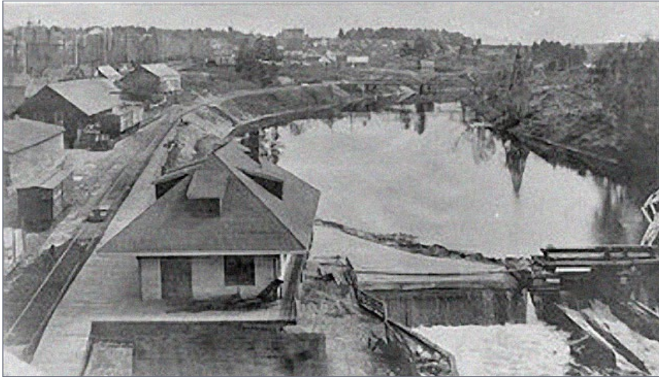
1. The station area of Pembroke, along the bank of the Muskrat River. The roundhouse is about ¼ mile down the track around the bend in the river. Author's collection
