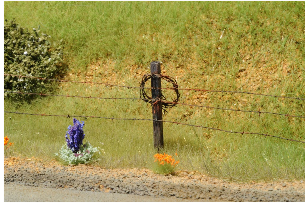
11. A view of a portion of the three-strand barbed wire fence with some extra wire stored for future field repairs when needed.
