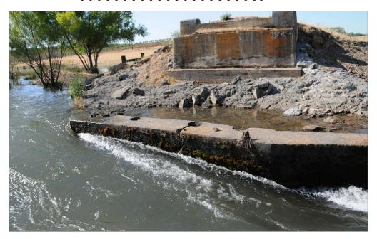
5. A current day view looking west shows an abutment and the pier for one of the trestle bents. The holes in the far side of the pier show that it was poured around the original driven-pile bent. That bent would have been sawed off after the new bent was in place.
