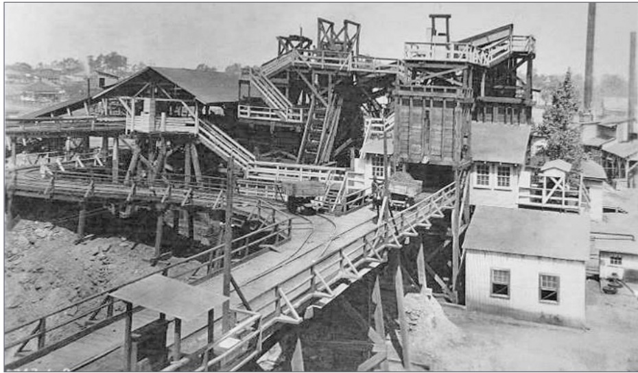
15. Pratt No. 5 tipple. In the background are the four-square company houses that were built by TCI. The beehive coke ovens are visible as well. John Stewart collection
