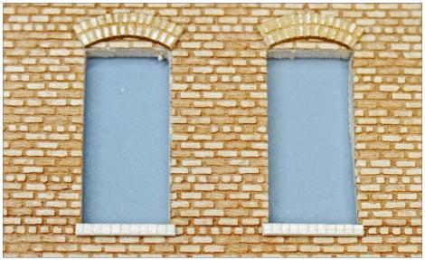
75-76. MMW manufactures two sizes of two-tier lintels – a small-radius 74LIN-HO (shown) and one with a large radius, 2TLIN-HO. Both are handled in the same manner. Place the lintel over the opening as shown, and cut the lintel at the point where it meets the corner of the opening. [76] shows the attached lintels and sills.
