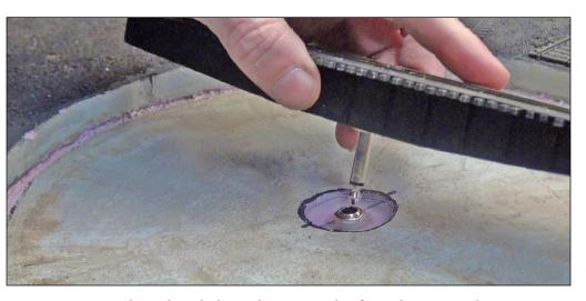
10. I cut a Plexiglas disk and centered a female microphone jack on it. This disk assembly was glued into the bottom of the pit to accept the male microphone jack attached to the turntable, as you see here.
