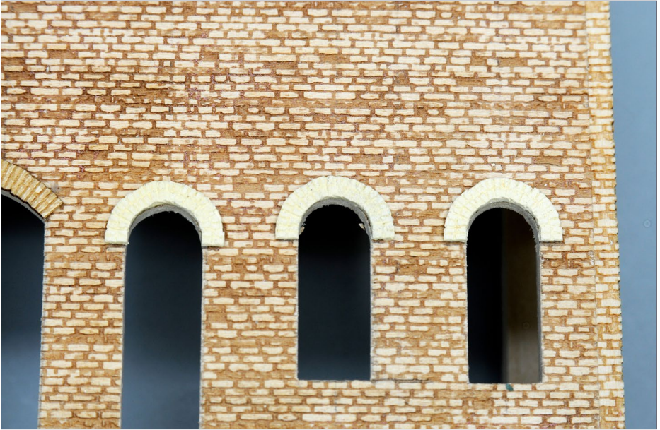
79. The cast lintels are applied above the window and personnel door openings. A small portion of the re-curved freight door lintel can be seen on the left.
