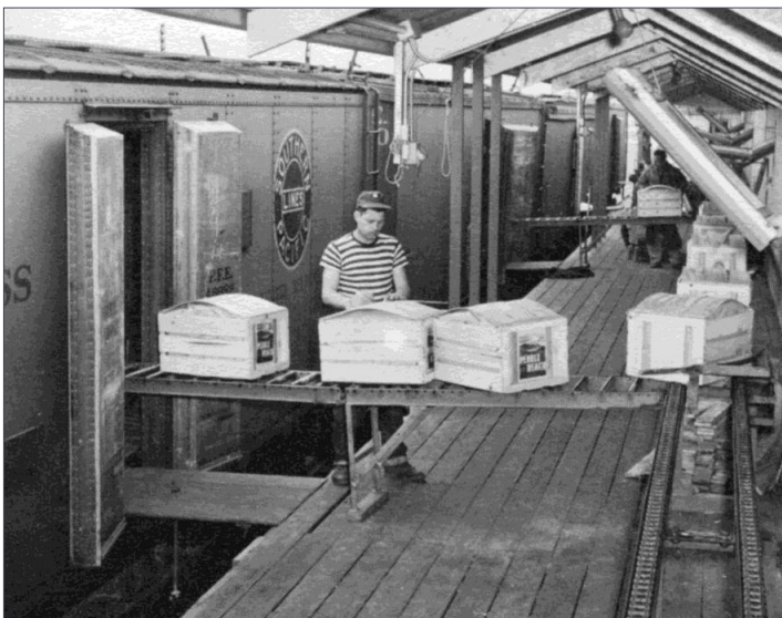
39. Note the clearance needed between the loading dock and car to safely open swing doors.
