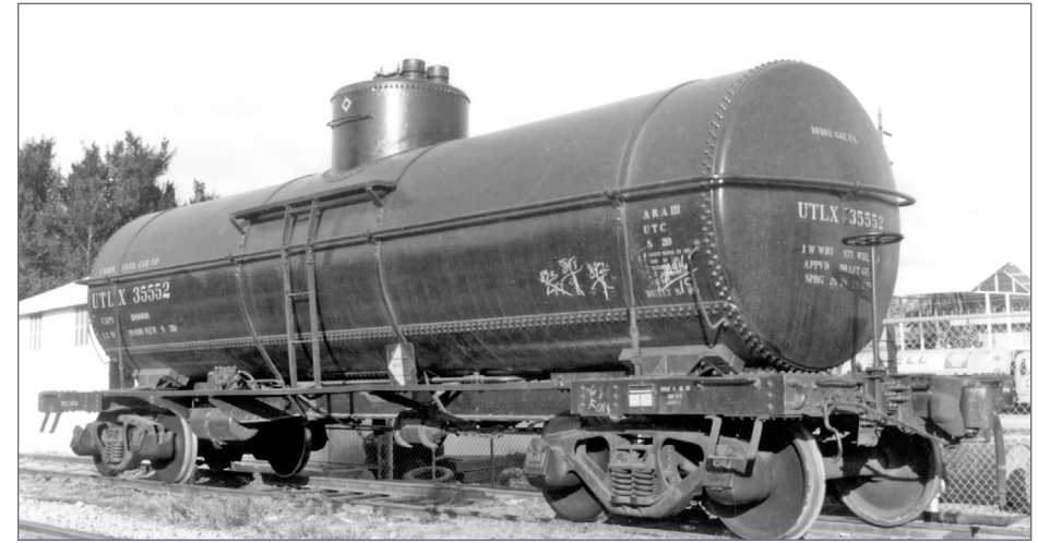
35. This UTLX tank car, photographed in 1948 and still showing (correctly) its “ARA Spec III” designation, has a standard “EMPTY” placard, the vertically divided diamond in black and white. Note the chalk marks on the car. The UTL car design has side and end sills of inward-facing channels, instead of the outward-facing channels of the AC&F underframe (Richard Hendrickson collection)
