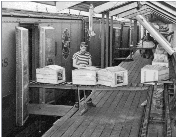
39. Note the clearance needed between the loading dock and car to safely open swing doors.
