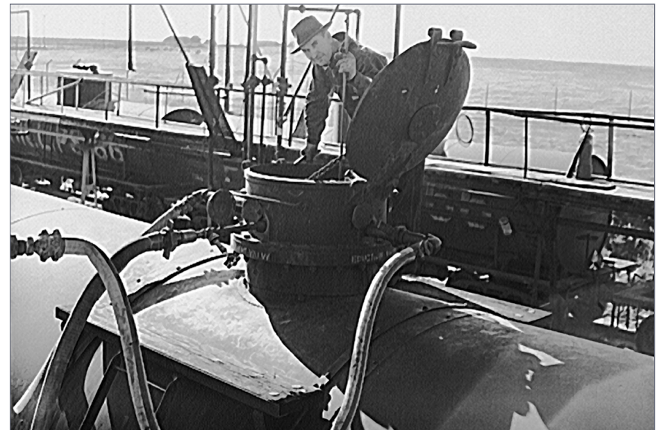
20. Unloading view of a high-pressure car. Pipe connections on sides of valve bonnet are evident. John Vachon photograph, 1943. (Library of Congress, negative LC-USW3-010341-D)
