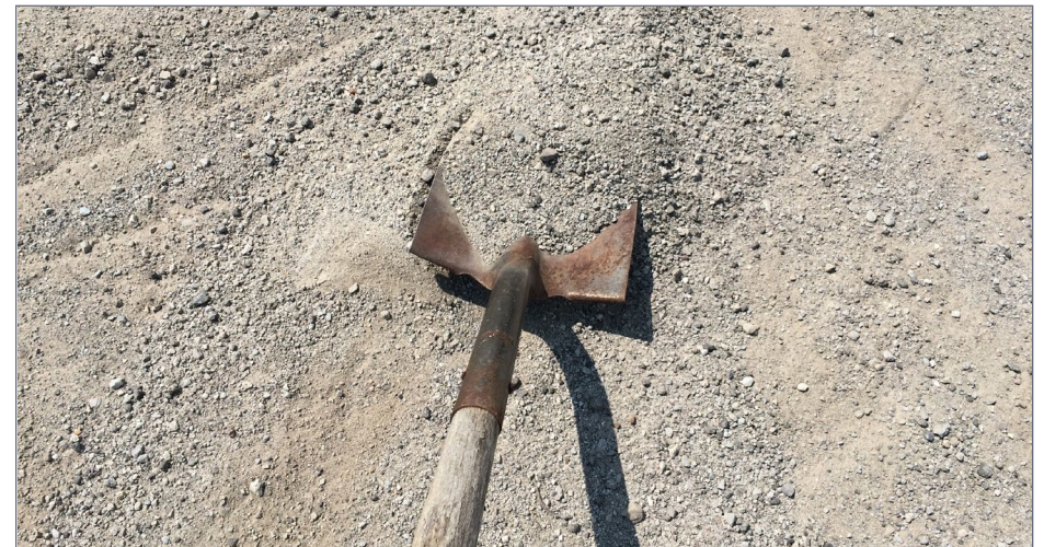
4. Scraping the top layer of gravel.
