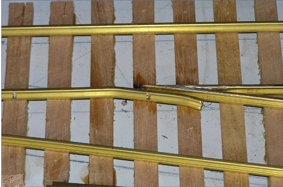
14. The straight closure rail is spiked in place.
