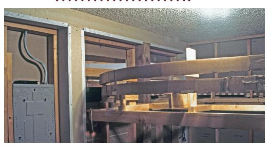
16. Here's the 40-inch radius helix in my workshop that replaced the 24-inch radius helix. This much larger helix with a 1.75 percent grade operates far better than the other helix – the difference is like night and day. The cardboard along the outside protects derailing equipment from heading toward the floor, although derailments in the helix have been quite rare.
