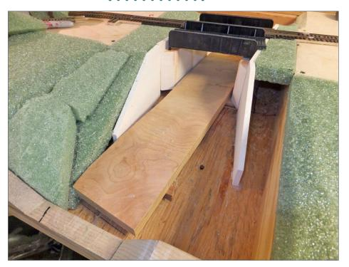
80. A new piece of plywood is installed to the proper height and will form the stream bed base. I don't like to use foam under Enviro-Tex as I've heard it can out-gas and cause bubbles. True or not, why take the chance?
