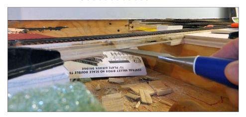
62. I wanted this bridge to capture the feel of the prototype through girder bridge. To have the girders high enough to look "right" to me, I decided to thin the subroadbed under the girders. I made saw cuts with a Japanese dovetail saw, and then chiseled out the area in between.
