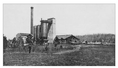
5. Woodward Iron Number 1 Furnace. Notice the resemblance to the Cranberry Furnace. Both furnaces were designed by the same individual in Pittsburgh, PA, as were other furnaces at the time. They were modified only to meet the space requirements of the company they were designed for. Woodward Family papers, University Libraries Division of Special Collections, The University of Alabama. *John Stewart collection*.
