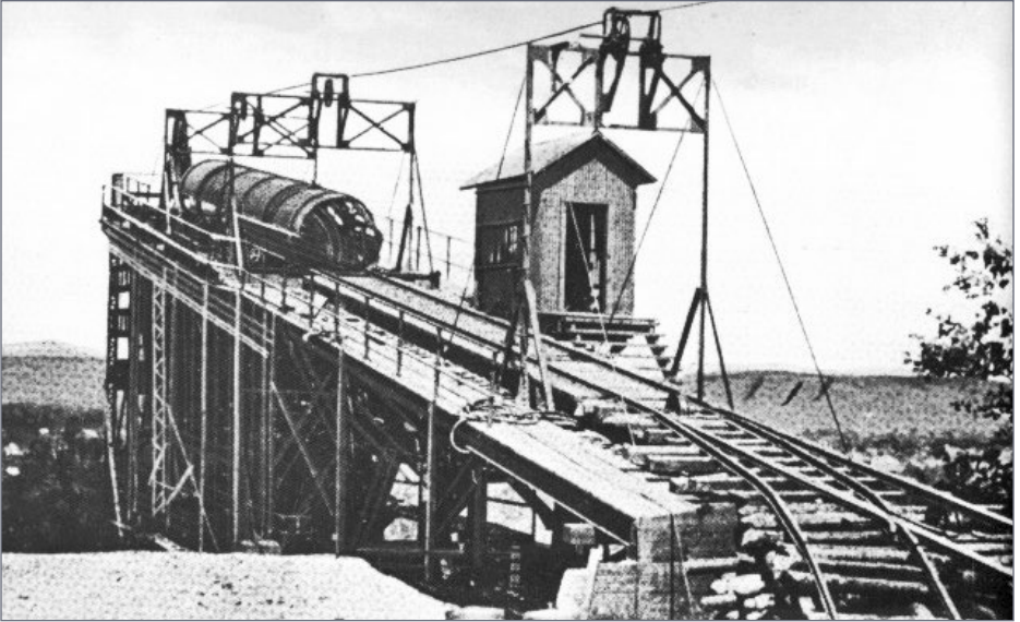
7. Woodward Iron tipple, either No.1 or No.2. Note the overhead cable sheaves that pulled the cars to the top of the incline for dumping. Photo from Mine, Mill and Microchip, a chronicle of Alabama enterprise , Wayne Flynt, Windsor Publications, 1987.
