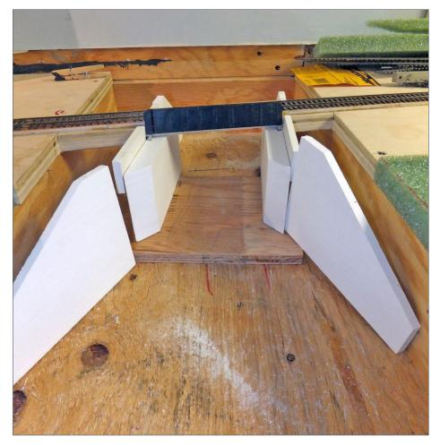
72. With the abutments in position, it was time to determine the nature of the wing walls and their positions.
