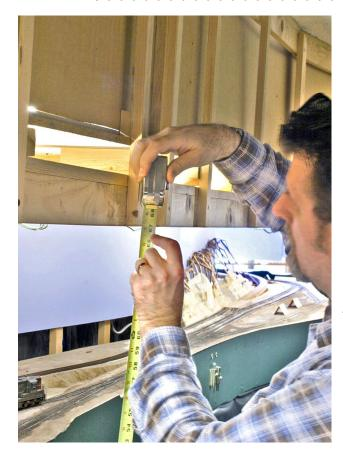
12. By testing with mock-ups first, I determined the best height for the bottom back edge of my upper deck benchwork was at the end of mu nose, which comes to 67 inches from the floor. This allowed me to see the lower deck all the way to the backdrop just fine, but kept the lighting out of sight. With the lower deck at 54 inches from the floor, this gave me a deck separation of 13 inches.
