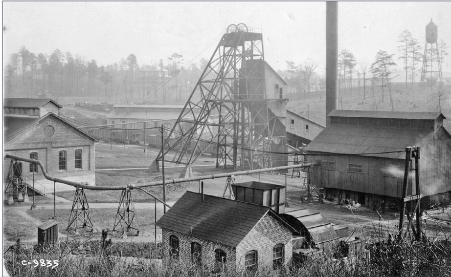
6. Prototype Mulga Mine. There is a lot of good modeling information in this photo. Note the blower house in the front of the photo, and the steam pipe running from the boiler house to the hoist house. Woodward Family papers. University Libraries Division of Special Collections, The University of Alabama. *John Stewart collection*
