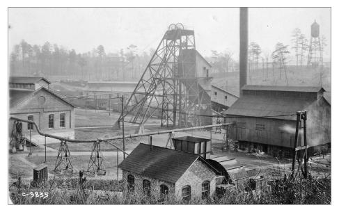
6. Prototype Mulga Mine. There is a lot of good modeling information in this photo. Note the blower house in the front of the photo, and the steam pipe running from the boiler house to the hoist house. Woodward Family papers. University Libraries Division of Special Collections, The University of Alabama. *John Stewart collection*
