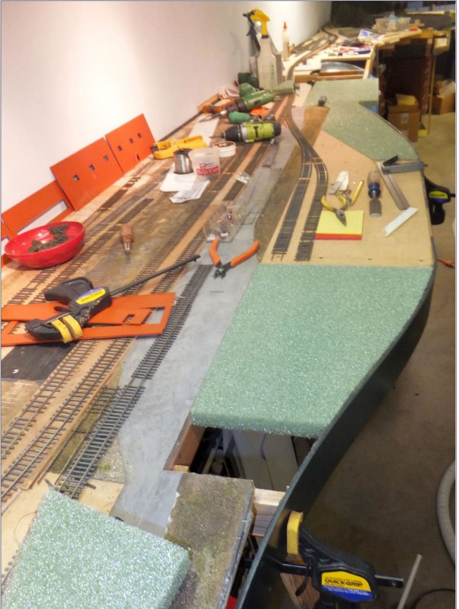
49. This elevated view shows the process of cutting and fitting florist's foam for the fill-ins.
