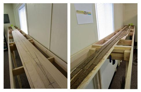
8-9. Laying out the track centerlines on the plywood, and then gluing down the cork roadbed.
