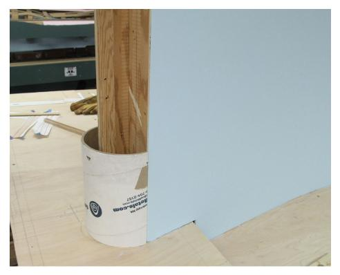
9. To tell the truth, I wasn't convinced we'd end up with a usable bullnose. You can see here that it did work – we placed one of the cut off ends of the bullnose against the mounting plate and it was less than 1/32" wider than the mounting plate on both sides. I can tell you this was a big relief!
