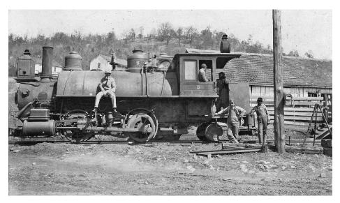
6. Woodward #5 an 0-4-2T. It looks like the trailing truck was an afterthought from the spacing under the engine. *John Stewart Collection*
