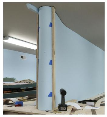
11. Remember that the bullnose was slightly wider than the backdrop? After scraping off the excess adhesive that oozed out of the seams. we covered the joints with blue painter's tape and temporarily screwed two pieces of 3/4" x 3" plywood
