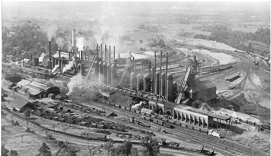
1. Aerial view of the Woodward Furnaces celebrating 75 years of service by the Southern Railway. From an article published in January, 1959 Ties The Southern Railway Magazine , and posted on southern.railfan.net .
