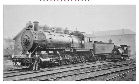
2. The engine on the right is one of the H. K. Porter 0-4-2Ts, either the #2 (Built June, 1882, construction # 498) or the #6. *John Stewart Collection*
