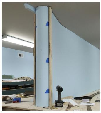
11. Remember that the bullnose was slightly wider than the backdrop? After scraping off the excess adhesive that oozed out of the seams, we covered the joints with blue painter's tape and temporarily screwed two pieces of 3/4" x 3" pluwood
